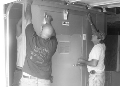
Installing New Walk-in-Freezer
