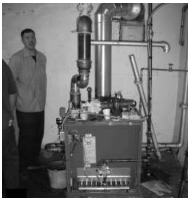
Work completed by: A & S Plumbing
